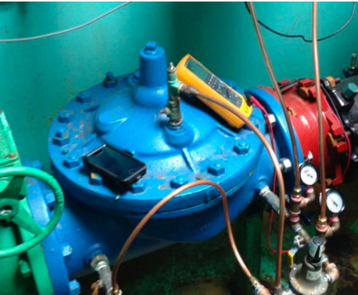
Figure B-2. Sample Pressure Reducing Valve (PRV)
